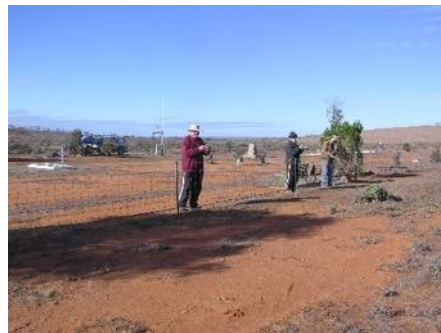
Ian Husband, Rod Lawrence and Barry Kakoschke fixing the anti-roo plastic tubing onto the top wire of the cemetery fence. You beauty, it works.
