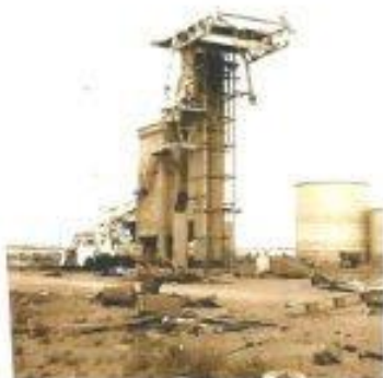
The once striking Main Shaft head frame partly demolished.
